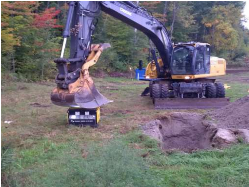
Fig. 5: GEM Mark 2 deployed on the Foundation Road Landfill Project, Chalk River
